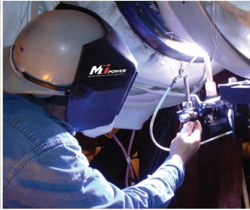
MTI welders operating orbital pipe welding equipment on site during the installation of the new steam chest.
