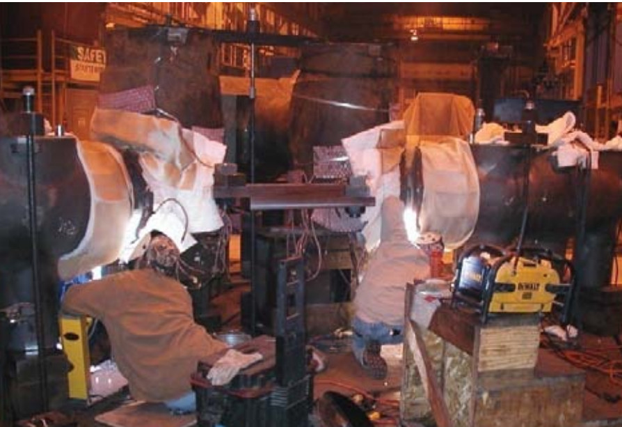
MTI welders operating orbital pipe welding equipment on site during the installation of the new steam chest.
