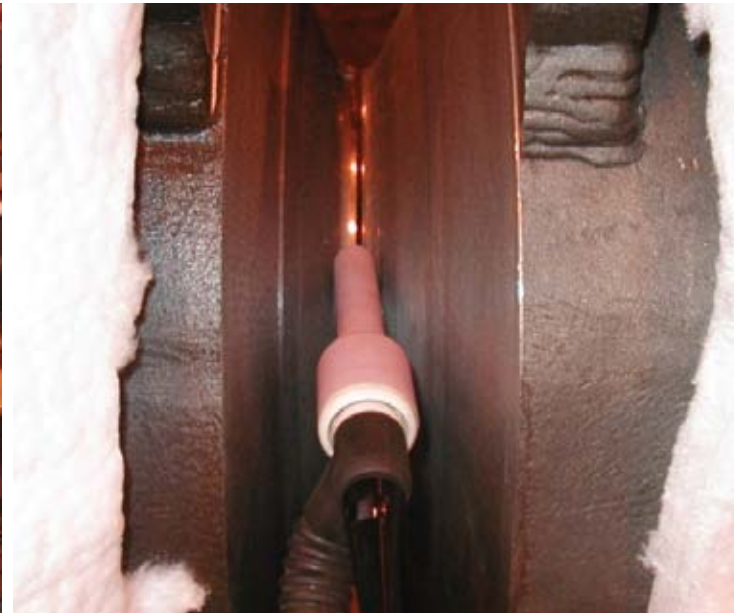
MTI welders operating orbital pipe welding equipment on site during the installation of the new steam chest.
