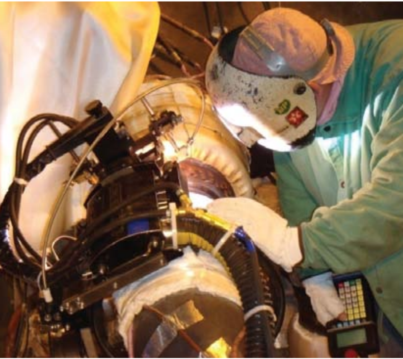
MTI welders operating orbital pipe welding equipment on site during the installation of the new steam chest.
